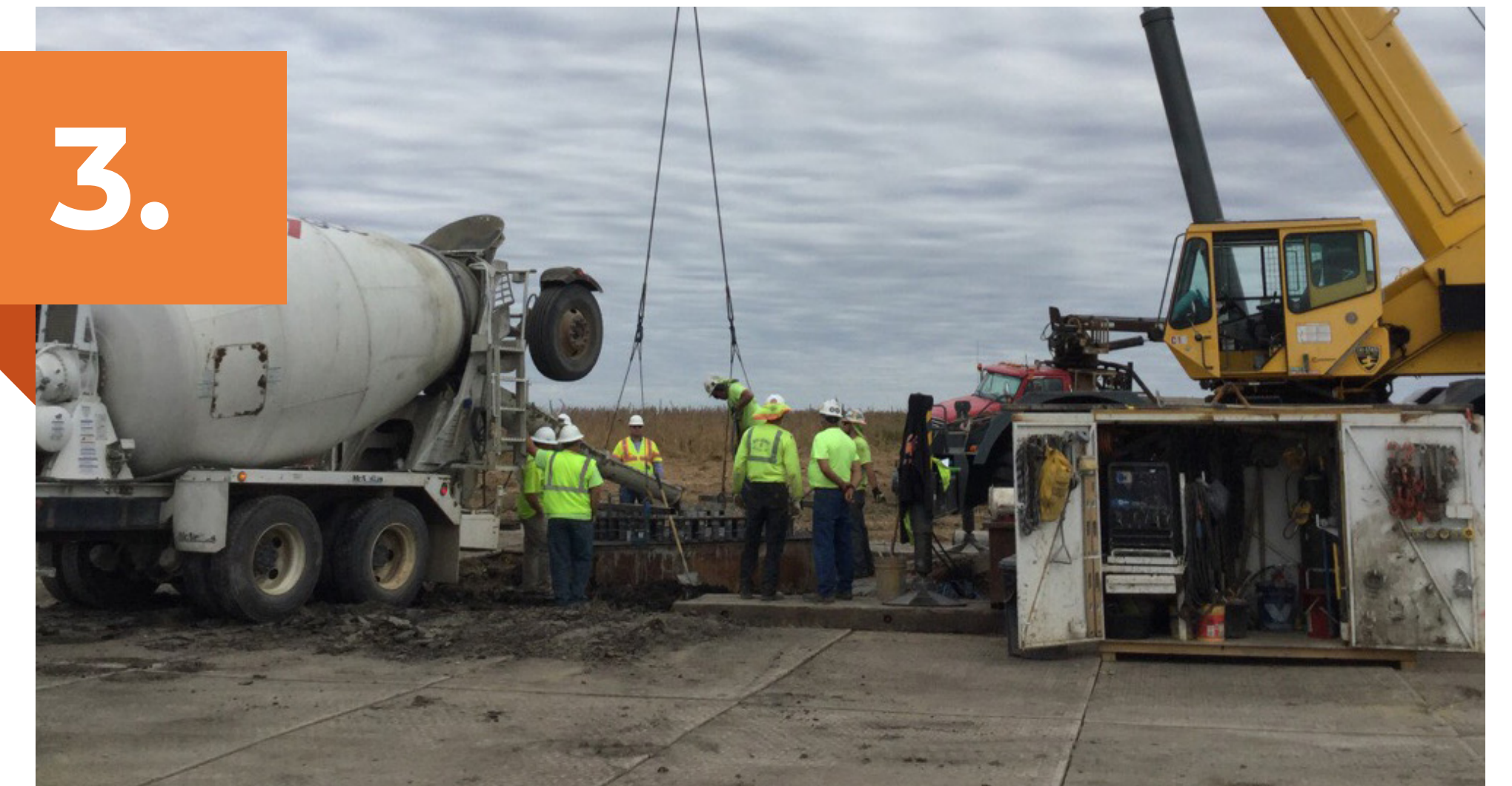
Foundation Drilling & Pouring
